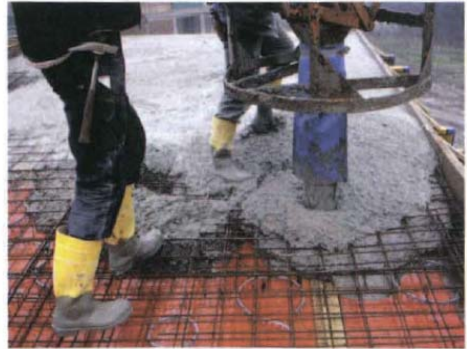
In-situ reinforced concrete being poured
