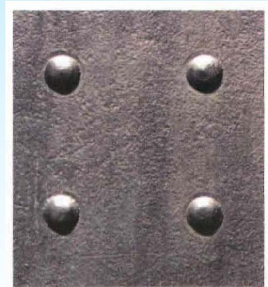
Solid rivets after installation
