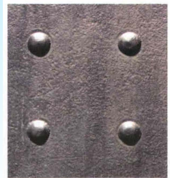
Solid rivets after installation
